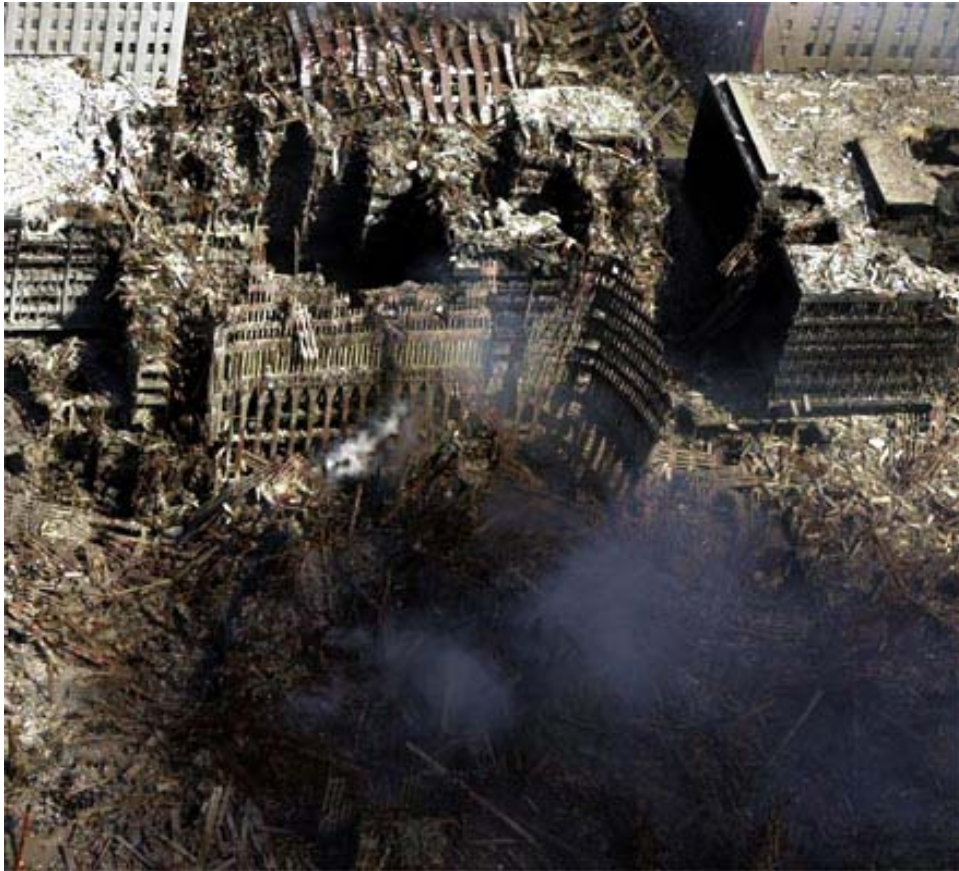
Figure 16 The material from WTC1 is essentially absent and the vertical holes cut through WTC6 can be seen. Note the absence of material in this void.
