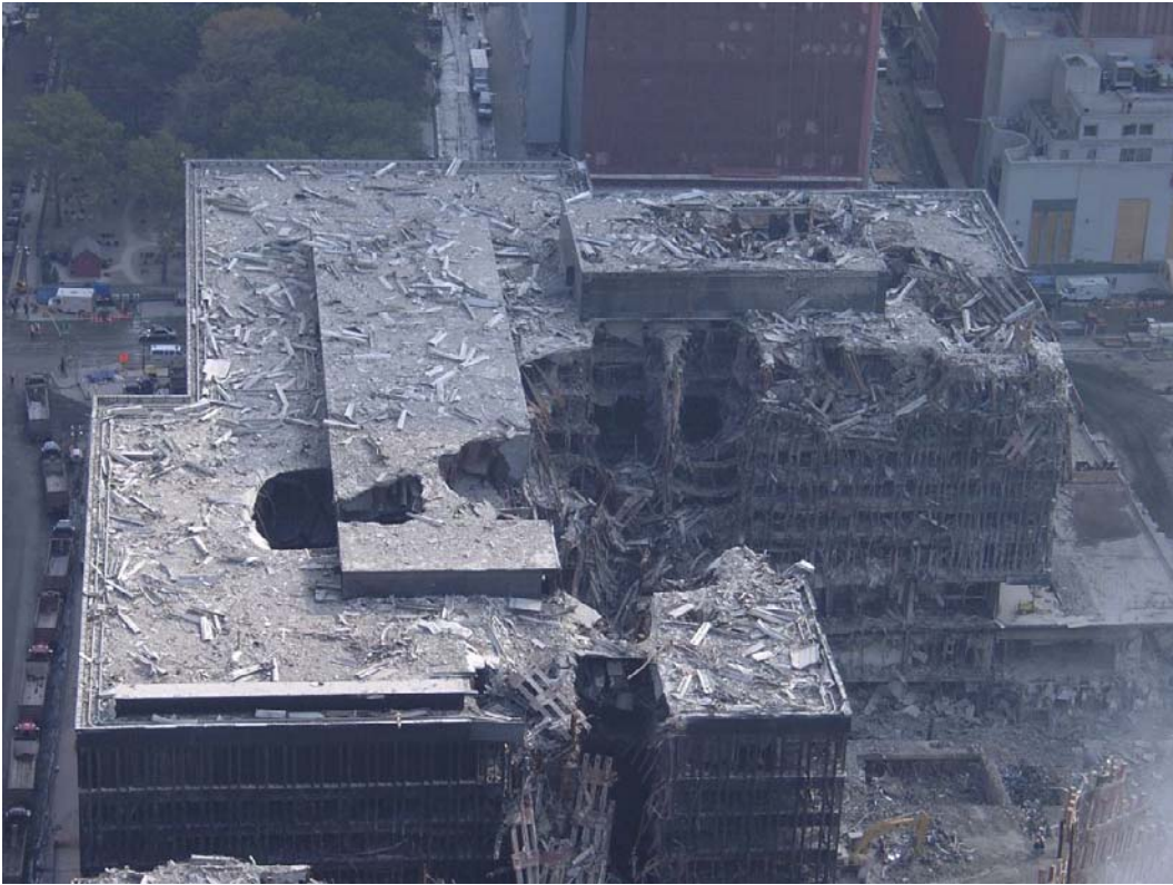
Figure 25 The perpendicular holes are found in several buildings and in the streets.
