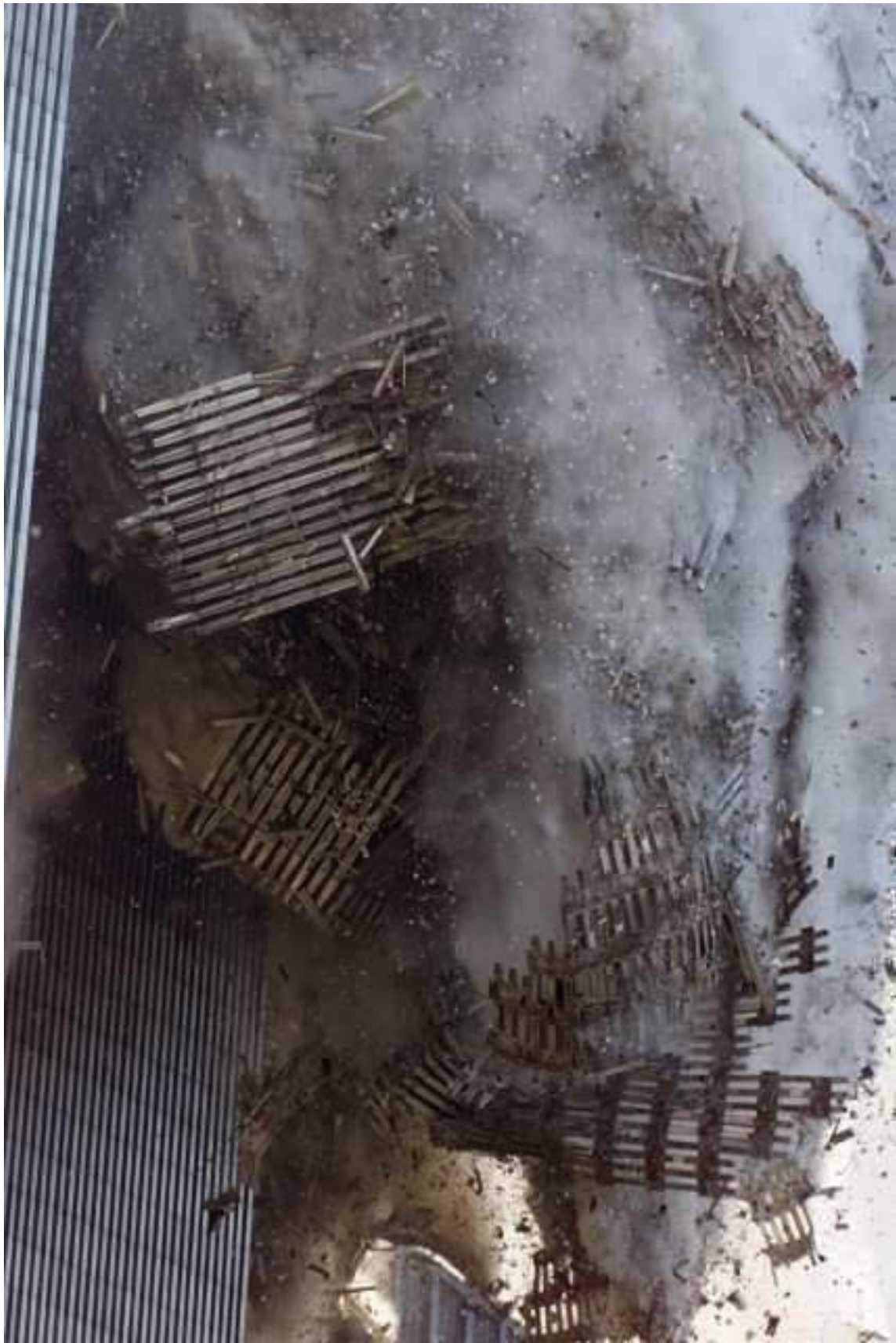
Figure 4 The steel is turning to dust as it falls.
