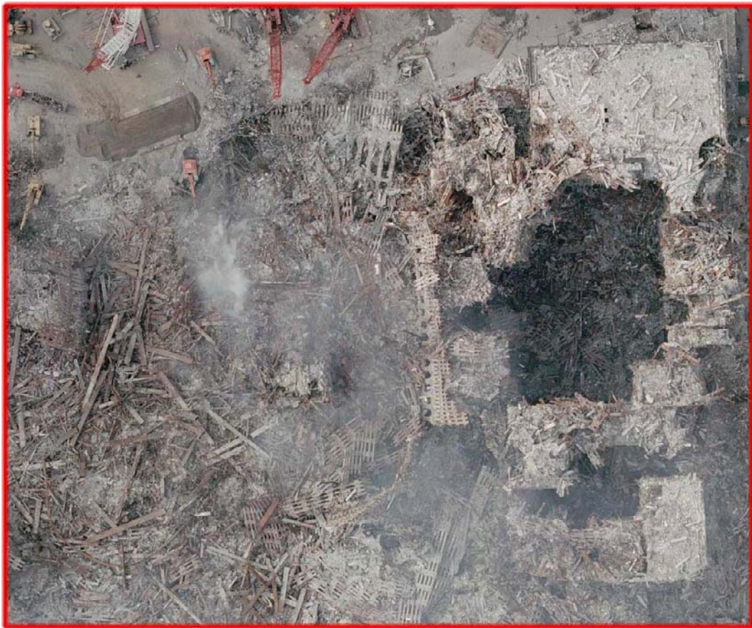
Figure 15 The remains of WTC6 are on the right and the footprint of WTC1 is on the left.
