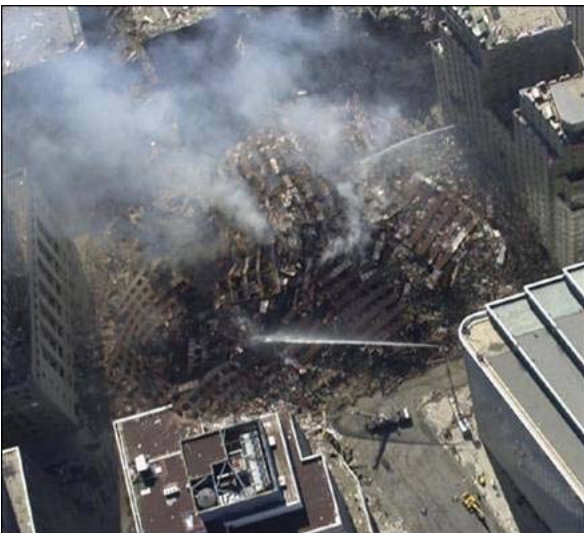
WTC 7 collapsed completely, onto its own footprint
