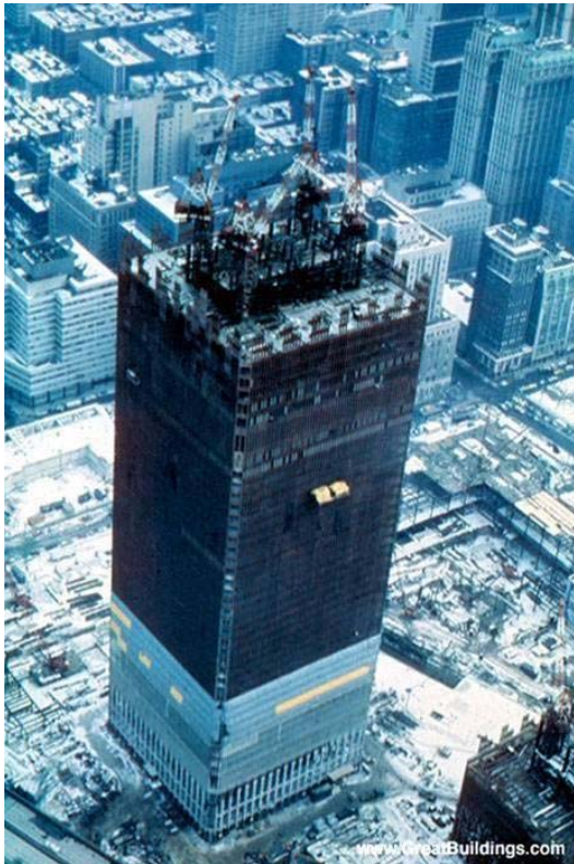
The WTC towers were solidly constructed with 47 steel core columns and 240 perimeter steel columns. 287 steel-columns total. Many doubt that random fires/damage could cause them to collapse straight down (official theory), and suspect explosives.
