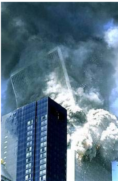
Top ~ 30 floors of South Tower topple over. What happens to the block and its angular momentum?
