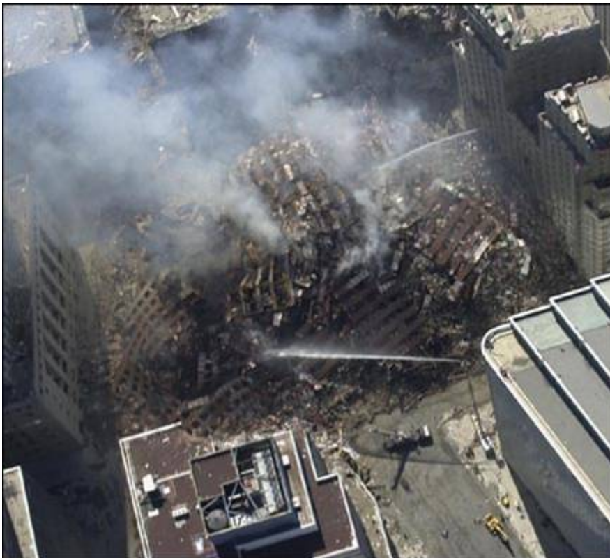
WTC 7 collapsed completely, onto its own footprint
