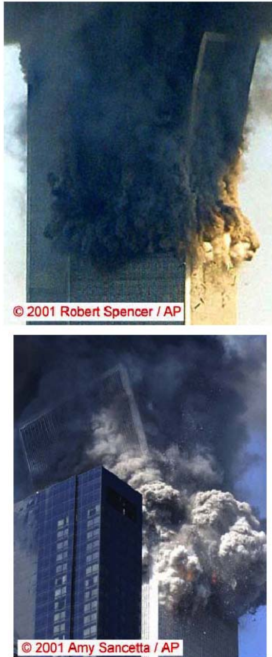
Figure 6–26. Kink on southeast corner near Floor 106 formed after collapse initiation.
