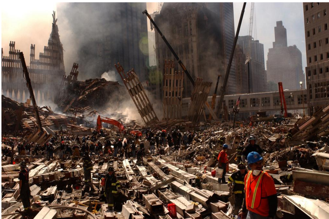
Figure 20. The remarkable "lay down" of steel wheatchex from the lower stories of WTC1 on West Street (West Side Highway). The WTC3 debris pile is in the background, next to the unsupported WTC2 wall. (9/13/01)
