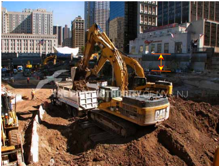
Figure 26. In September 2007, they are taking dirt out from the eastern bathtub. Where did the dirt come from? It was trucked in from outside Manhattan.
