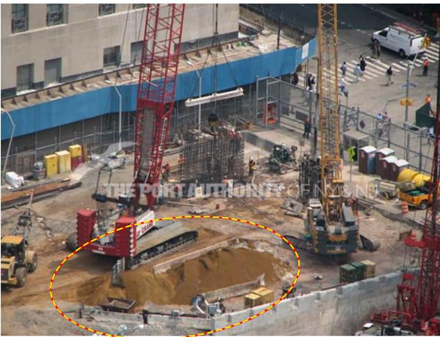
**Figure 28.** Dirt has been brought in to the east bathtub (August 2007).
