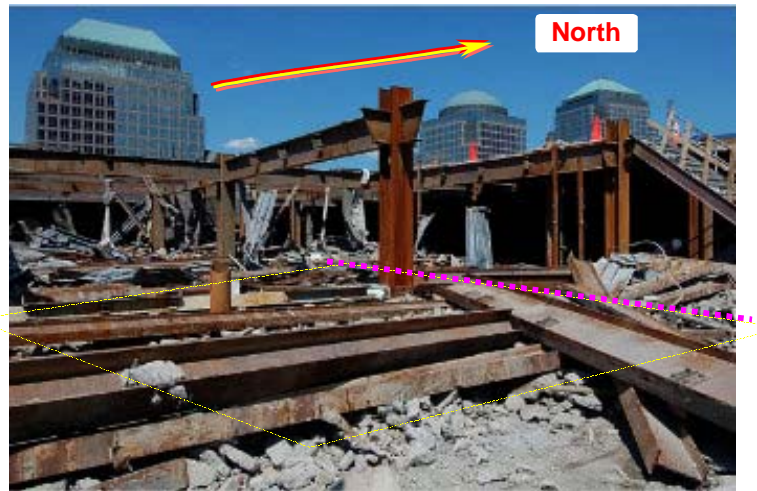
Figure 87. This is Bankers Trust being taken apart. Floors have been removed down to approximately the elevation shown in Figure 86. The very rusty beam (furry-rust) is approximately in the location shown in Figure 86. Recognize any "rustification" out there?
