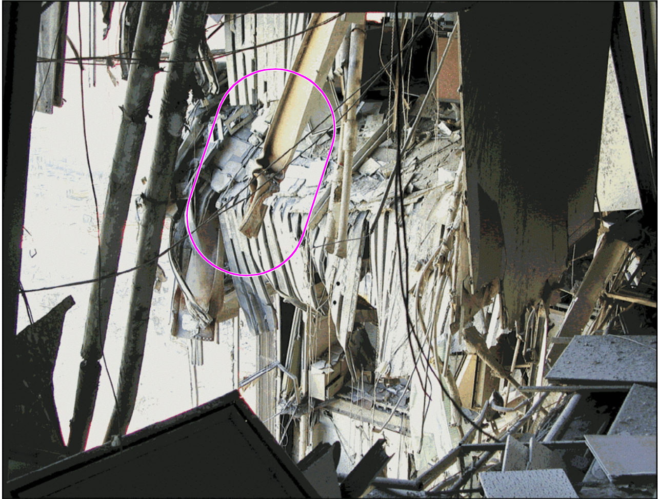
Figure 6-10 Area of collapsed floor slab in bays between C-8, E-8, C-7, and E-7, from the 15th floor.
