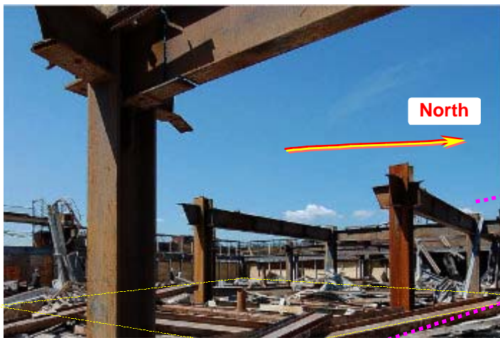
Figure 88. As more and more beams and columns are removed, what was once an enclosed building opens up to the sky.
