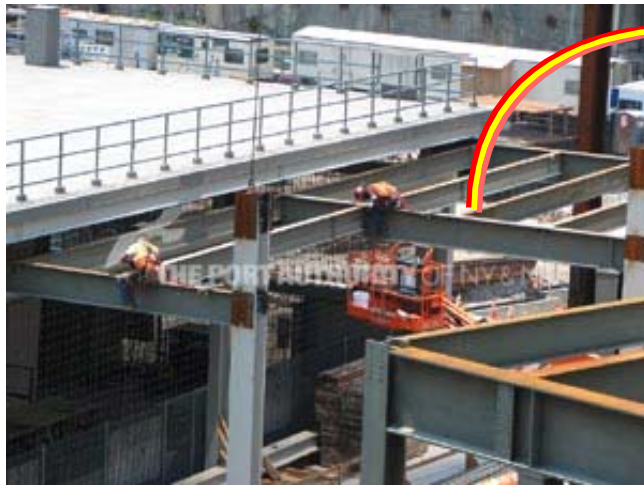
Figure 96. Beams rust before they are put in place. (06/07)
