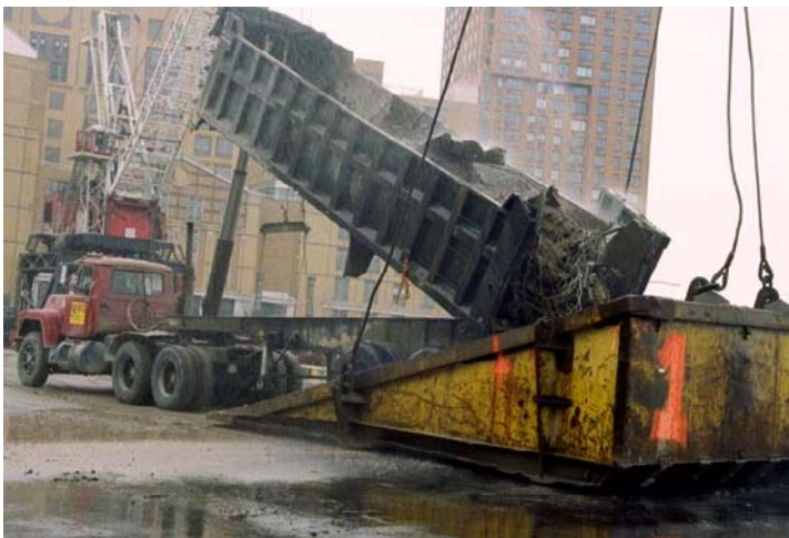
Figure 101. March 15, 2002, a truck dumps fuming dirt into the bucket of a 500-ton floating crane located at FEMA's Pier 25 loading site, a few blocks north of Ground Zero. The fuming dirt is sprayed with water. (3/15/02)
