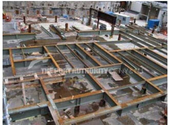
Figure 95. Rust appears very quickly in some areas and not others. (06/07)
