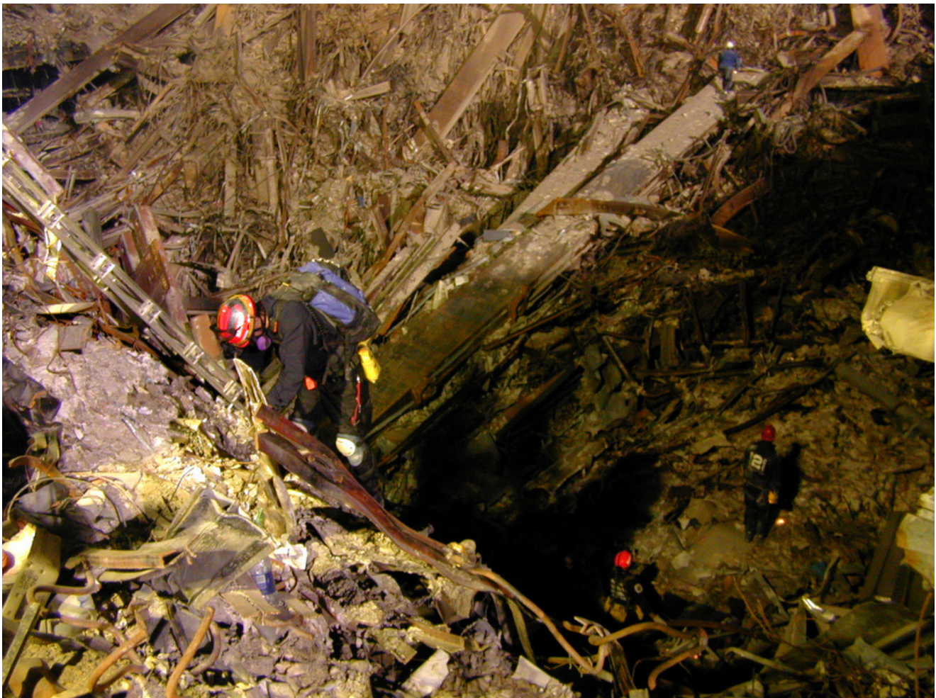
Figure 17. GZ workers descend into the subbasements below WTC2. While there is extensive damage, there is little building debris at the bottom of the hole. There is no sign of molten metal. A worker in the distance walks along a massive core column. There is little to no material in these holes. (photo filed 9/18/01)
