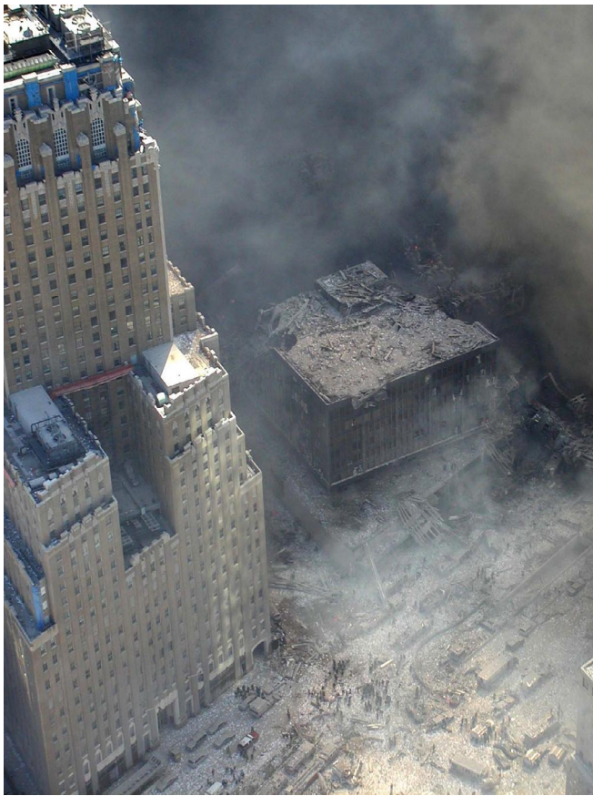
Figure 30. Looking southeast toward WTC6, across the West Street and Vesey Street intersection.
