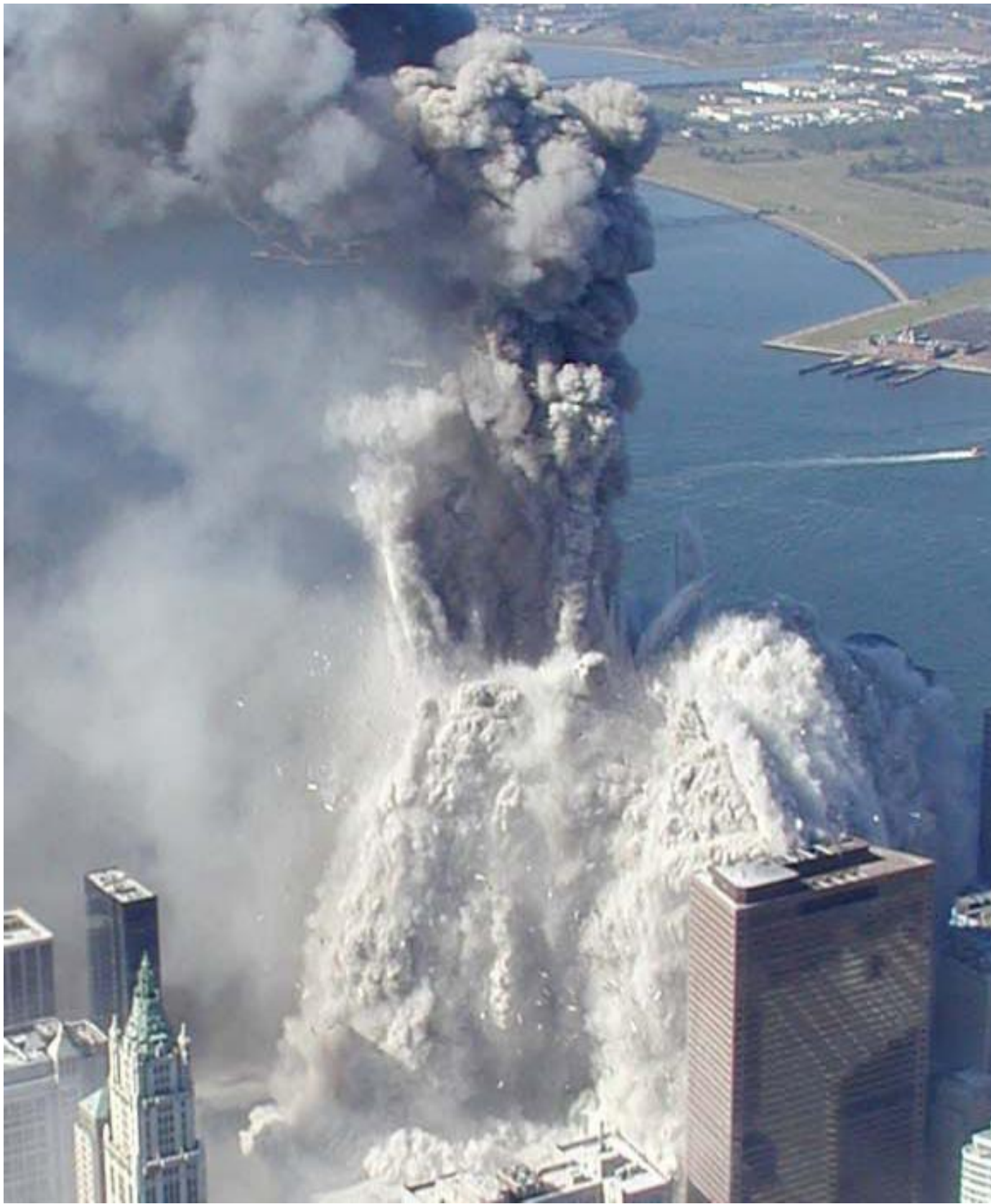
Figure 66. This is not a collapse and it is fraudulent to have so stated. This may be evidence of criminal intent to deceive the public. It is also evidence of the use of DEW. No other explanation fits the depiction of destruction seen above as well as that of use of DEW.
