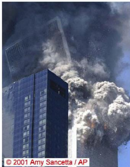
Figure 6–26. Kink on southeast corner near Floor 106 formed after collapse initiation.
