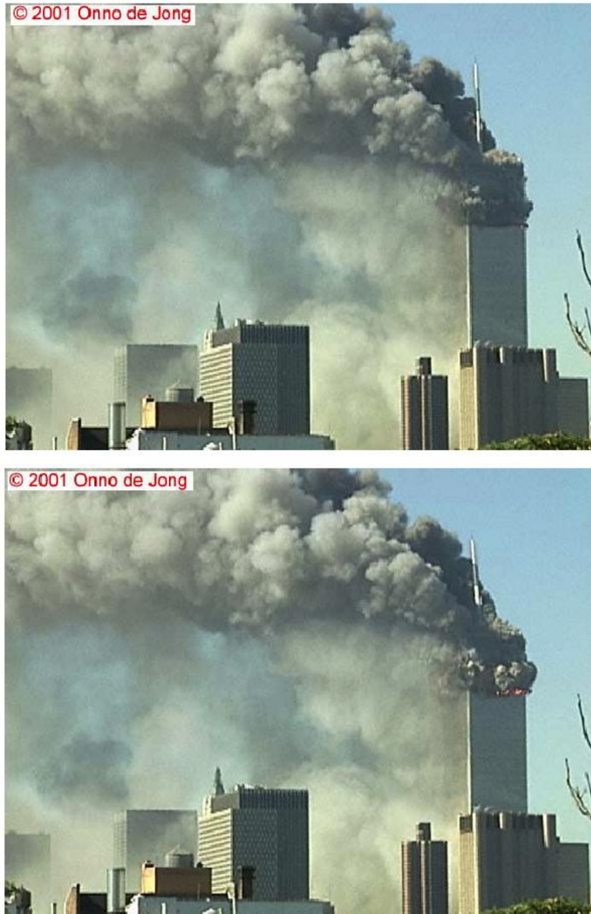
Figure 6–9. Smoke expulsion at Floor 98 from north and east faces at collapse initiation.
