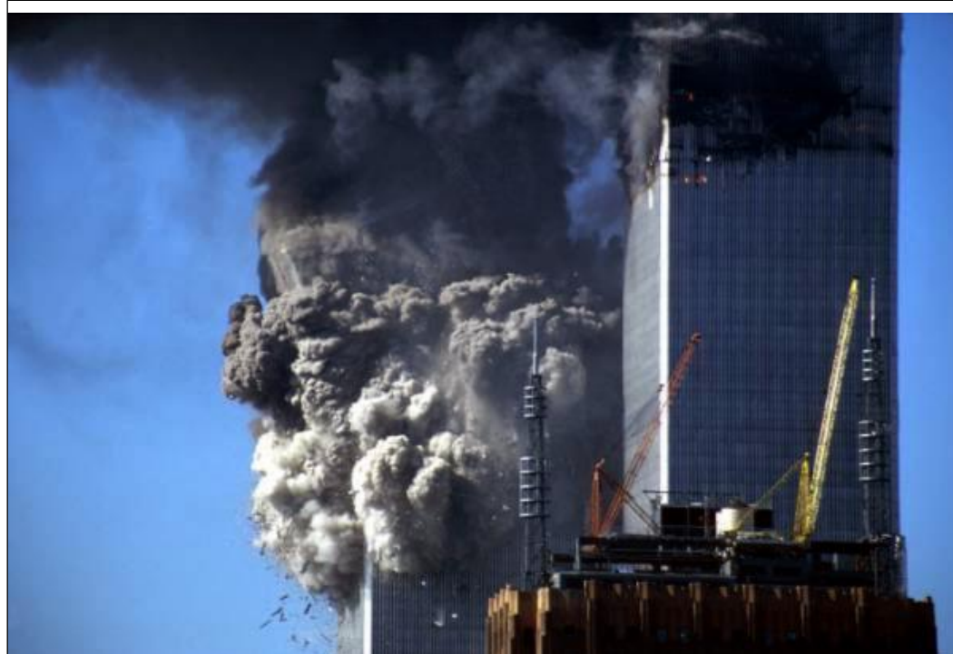
Figure 13. WTC2 tipping eastward, as viewed from the north. The tipping top is disappearing
