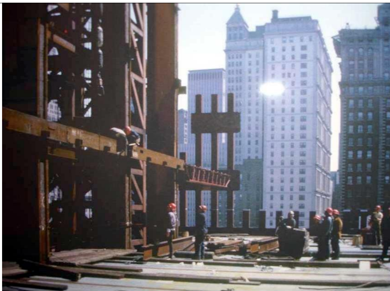
Figure 1. The massive core columns of the WTC, as seen during construction, Because of their mass, they would be an enormous heat sink.
