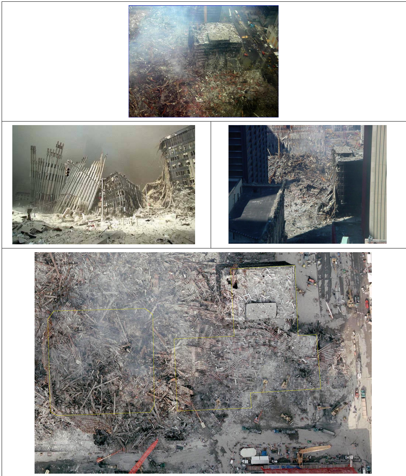
Figure 15. WTC4 footprint at the bottom, the remaining WTC4 north wing on the right, and the WTC2 footprint above.
