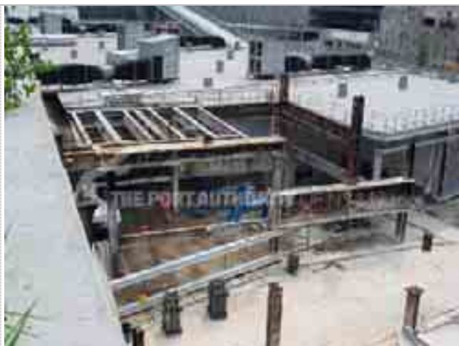
Figure 67. New beams rusted. June 2006 (6/?/06) Source: e 060600_RampJ02.jpg
