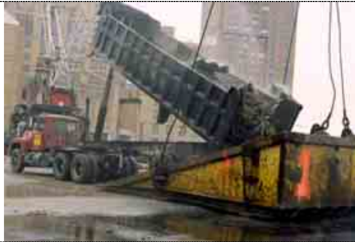
Figure 36. New York, NY, March 15, 2002 -- A truck dumps debris into the bucket of a 500-ton floating crane located at FEMA's Pier 25 Loading Site, a few blocks north of Ground Zero.
