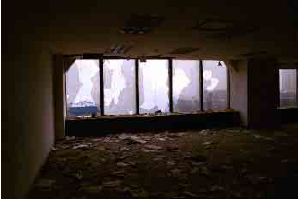
Figure 20. Round holes through glass, looking out of the One Liberty Plaza Bldg., over the remains of WTC4 and WTC5, with WTC2 in the distance, viewed through the far-left window. There are no large pieces of broken glass visible on the floor. (?/?/01)
