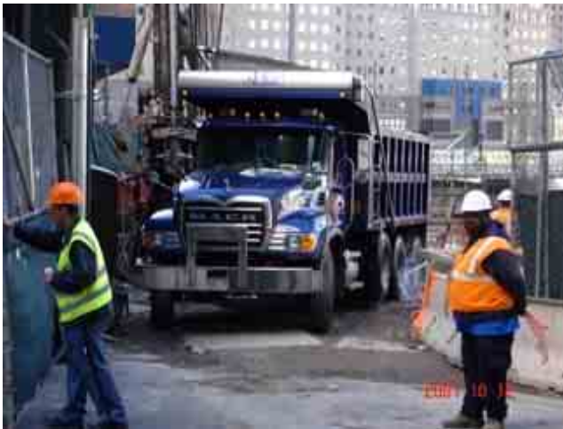
Figure 46. Dump truck being hosed down before leaving the site through the Liberty Street gate. (10/12/07)
