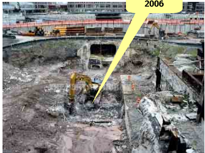
Figure 41. A view west along where the PATH train tracks were. Stirring the mud triggers fuming. five years after 9/11/01.
