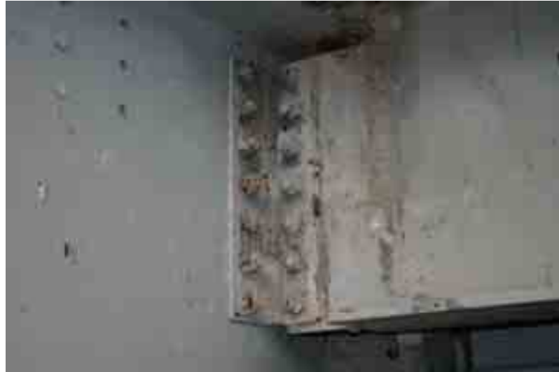
Figure 86. This beam was painted in June 2007. (10/09/07) Source
