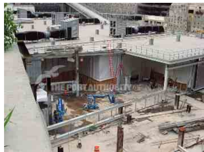
Figure 68. Infected beams removed, probably within days.
