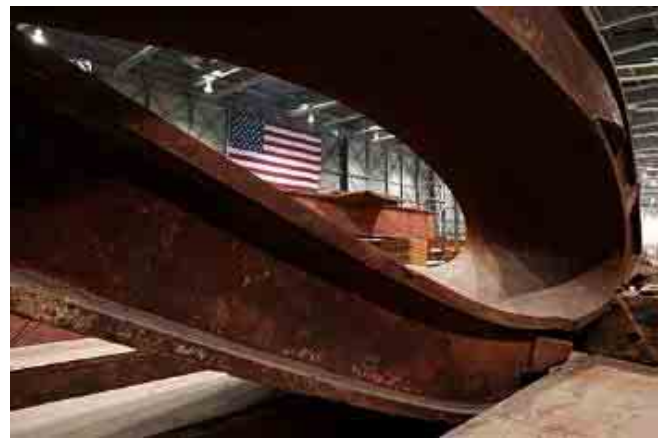
Figure 116. Buckled beams, characteristic of a gravity-driven collapse, were virtually non-existent at the WTC site. This bend is greater than 180°. (2002)
