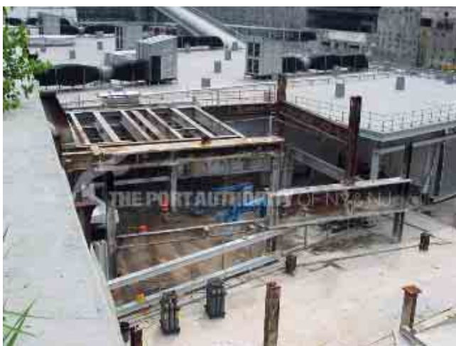
Figure 67. New beams rusted. June 2006 (6/?/06)
