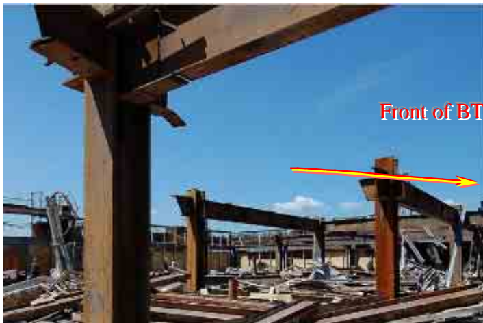
Figure 63. As more and more beams and columns are removed, what was once an enclosed building opens up to the sky.
