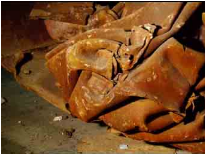
Figure F-A-2c: Collapsed part of Column 210.
