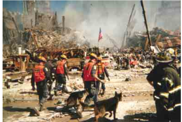
Figure 90. More rust (9/13?/01) Source:
