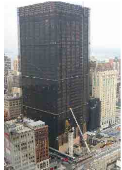
Figure 53. The structural and cosmetic damage to the building has been rehabilitated. (07/28/06)
