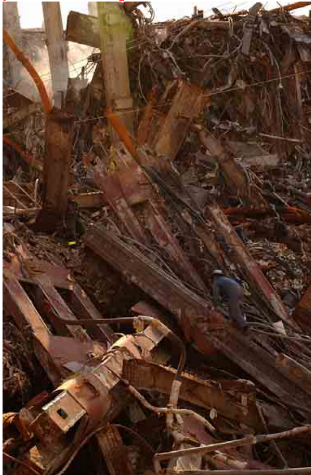
Figure 94. Original photo. It appears that pipes either rusted a lot or not at all. (9/16/01) Source
