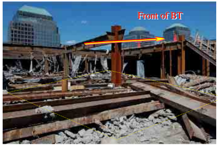
Figure 62. This is Bankers Trust being taken apart. Recognize any "rustification" out there?
