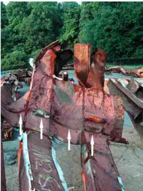
Figure 159. WTC beams (9/05): NCSTAR1-3c-P197_cc.jpg
