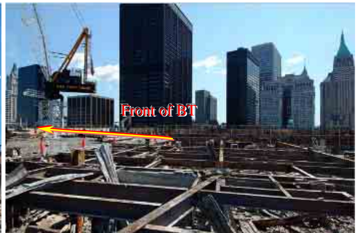
Figure 64. Once the concrete slab and metal decking are removed, what remains is a steel skeleton of each floor. There is little rust in the southwest corner of the building, even though it is open during the deconstruction from the top down.
