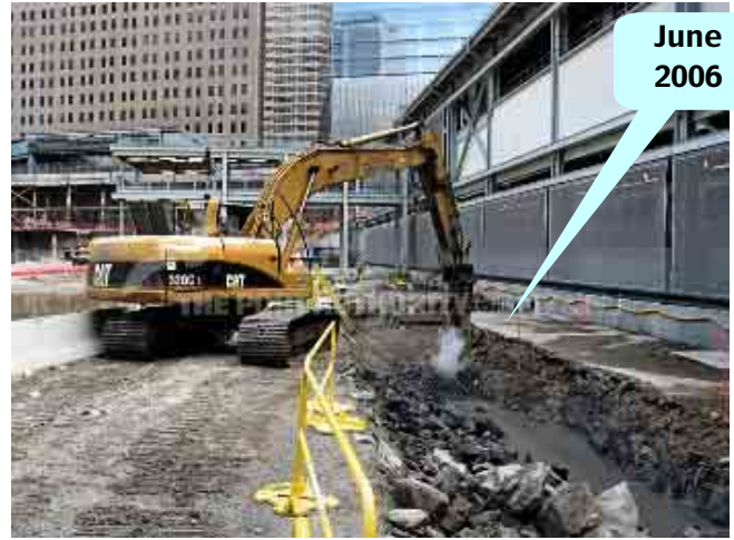
Figure 37. June 2006, looking north in the big bathtub. The new WTC7 is in the distance, on the right. Here's why the dirt is needed. This is the same "puff-ball poofing" we saw in October! (6/06)
