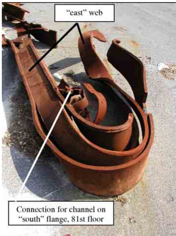
Figure 143. "Jellification" of WTC core columns.
