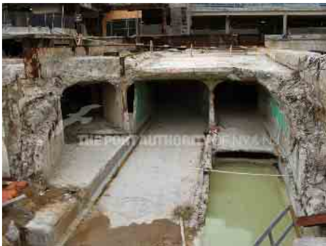
Figure 40. A view east where the PATH tracks were. Note, this area was not filled with dirt. The water here looks like what is seen in a typical rock quarry, not a muddy construction site.
