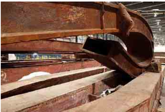
Figure 115. WTC core column curled, not buckled. A gravity-driven "collapse" would not do this. The beam above has smooth curves, without kinks. (2002)
