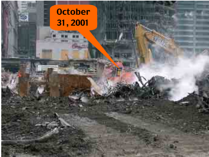
Figure 42. Fuming emerges from the wet dirt in the area between where WTC2 and WTC4 once stood. (10/31/01)
