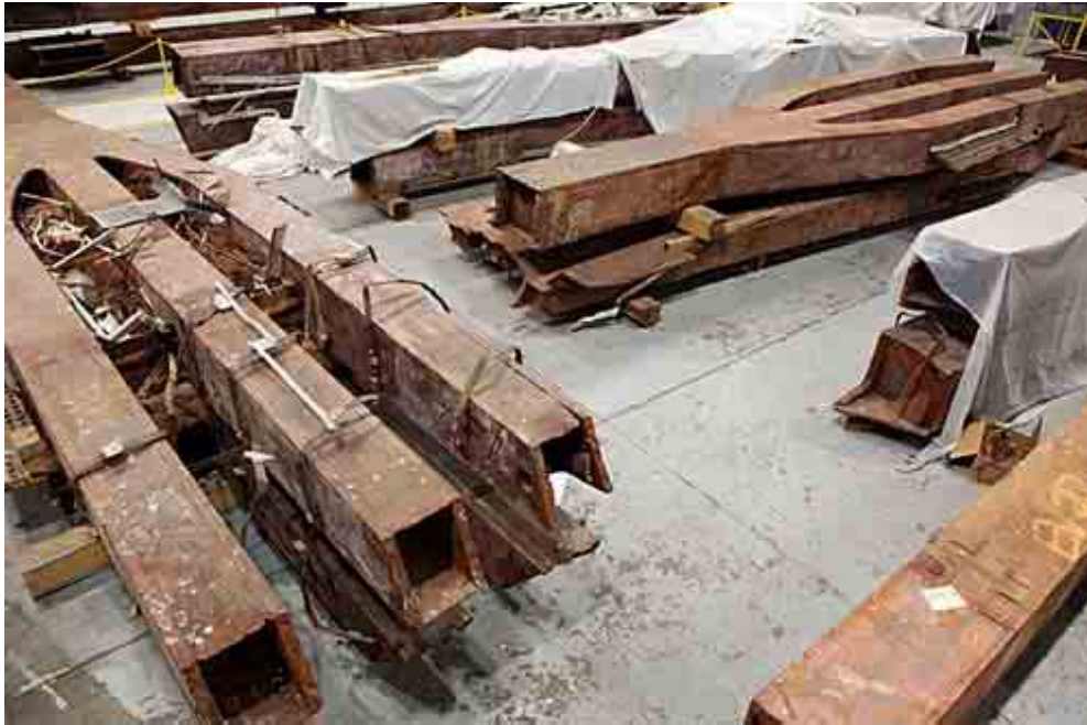
Figure 148. These columns don't look like 500,000 tons of building landed on them.
