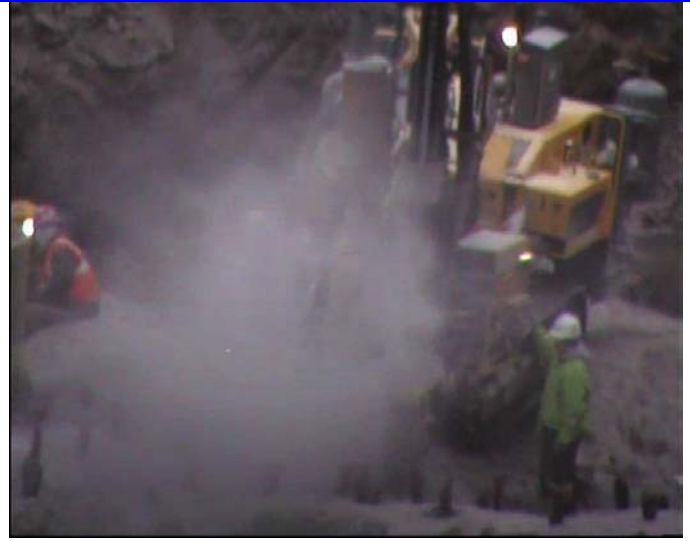
Figure 7. Digging stirs up fuming. (1/17/08) Source: Wood, Johnson,
