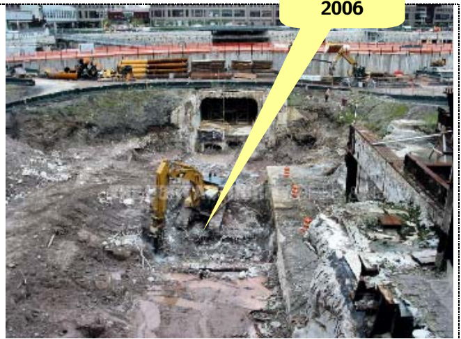
Figure 41. A view west along where the PATH train tracks were. Stirring the mud triggers fuming. five years after 9/11/01. (9/06)
