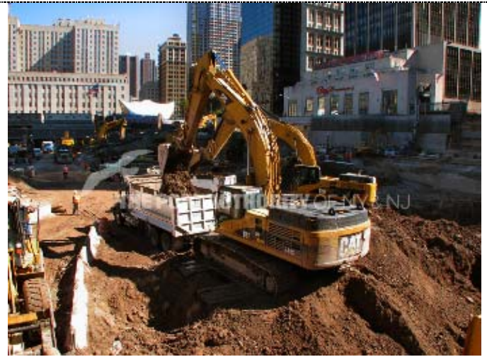
Figure 43. In September 2007, they are taking dirt out from the eastern bathtub. Where did the dirt come from? It was trucked in from outside Manhattan. (9/07)
