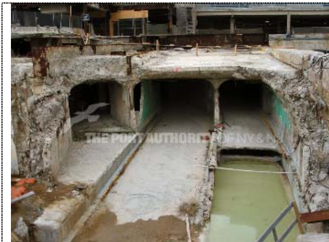
Figure 40. A view east where the PATH tracks were. Note, this area was not filled with dirt. The water here looks like what is seen in a typical rock quarry, not a muddy construction site. (4/06)
