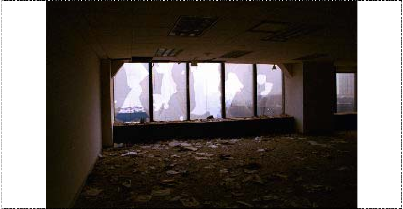
Figure 20. Round holes through glass, looking out of the One Liberty Plaza Bldg., over the remains of WTC4 and WTC5, with WFC2 in the distance, viewed through the far-left window. There are no large pieces of broken glass visible on the floor. (?/?/01)
