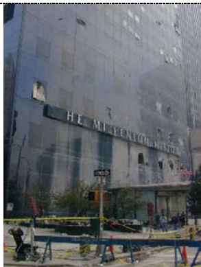
Figure 22. Few windows look damage on the front face of the Millenium Hotel one week after 9/11/01. (9/18/01)
