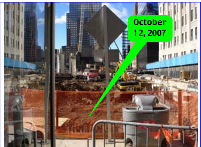
Figure 5. By three days later (Friday), most of that dirt pile is gone. (10/12/07) Source: Wood, Gerst, Reynolds
