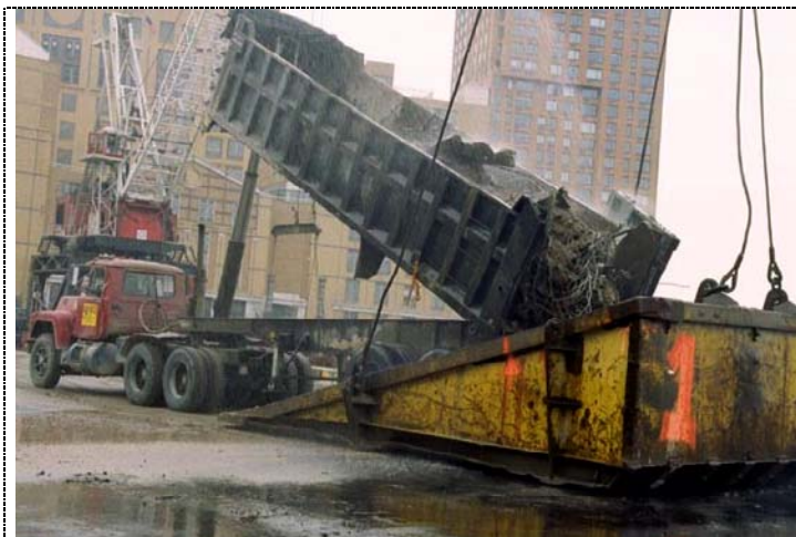
Figure 36. New York, NY, March 15, 2002 -- A truck dumps debris into the bucket of a 500-ton floating crane located at FEMA's Pier 25 Loading Site, a few blocks north of Ground Zero. (3/15/02)
