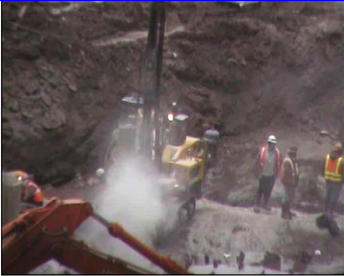
Figure 6. Digging stirs up fuming. (1/17/08) Source: Wood, Johnson,
