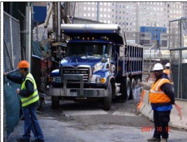
Figure 46. Dump truck being hosed down before leaving the site through the Liberty Street gate. (10/12/07)
