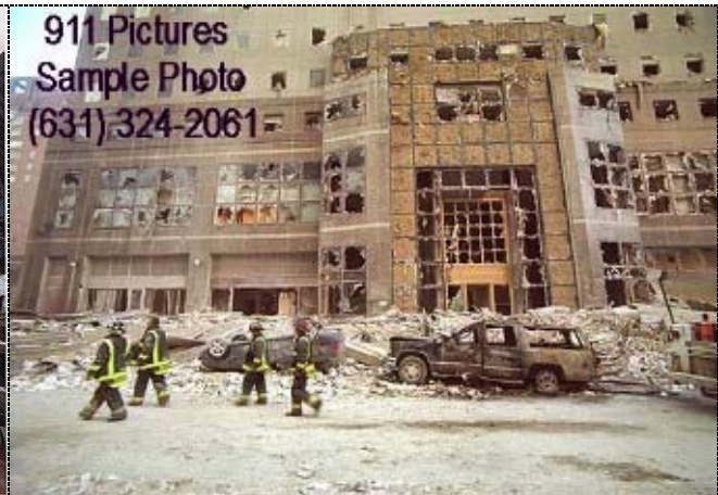
Figure 19. Flipped car in front of a damaged SUV, in front of WFC1. (9/12/01)
