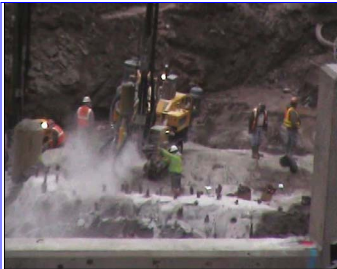
Figure 8. Digging stirs up fuming. (1/17/08) Source: Wood, Johnson,
