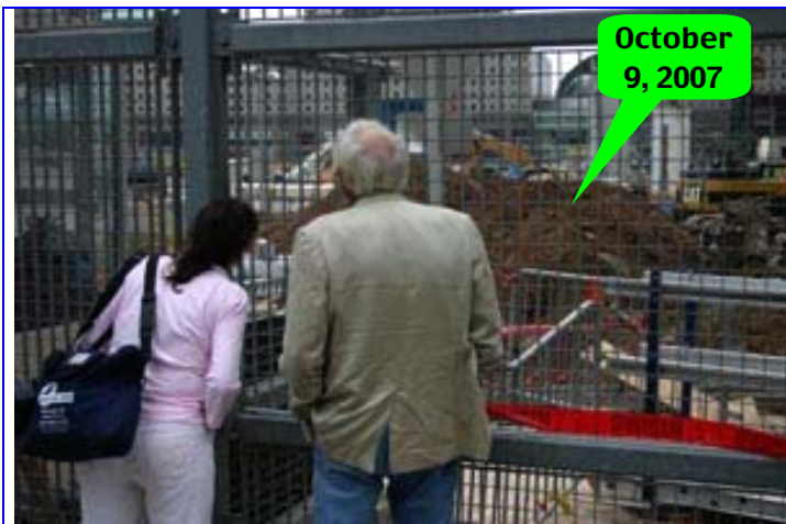
Figure 4. Looking west across the fresh dirtpile near Church and Vesey Streets. On Tuesday, there was a fresh new pile of dirt. It could have been potting soil or topsoil. Dirt is not used to make a new building foundation. (10/9/07) Source: Wood, Gerst, Reynolds
