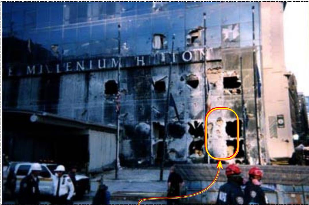
Figure 24. Round holes with no evidence they were caused by a projectile. To the contrary, the region noted above is unscarred behind the damaged glass façade. It is as if a big soldering iron made these holes and penetrated no further.
