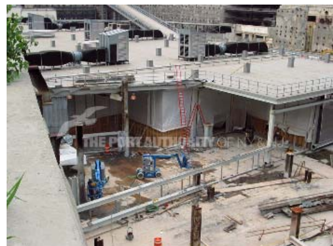
Figure 68. Infected beams removed, probably within days.
