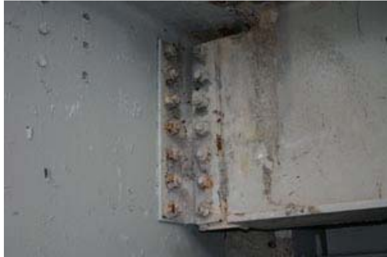
Figure 86. This beam was painted in June 2007. (10/09/07) Source
