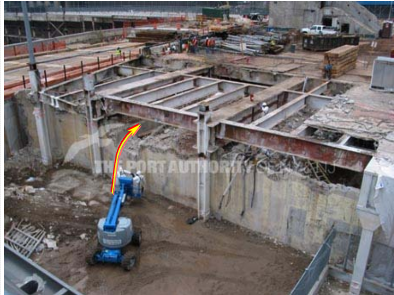
Figure 66. Why is this inspection being done with white hazmat suits? This is the area where the old PATH terminal was. 061200_HMdemo03.jpg (01/?/07)
