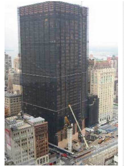
Figure 53. The structural and cosmetic damage to the building has been rehabilitated. (07/28/06)
