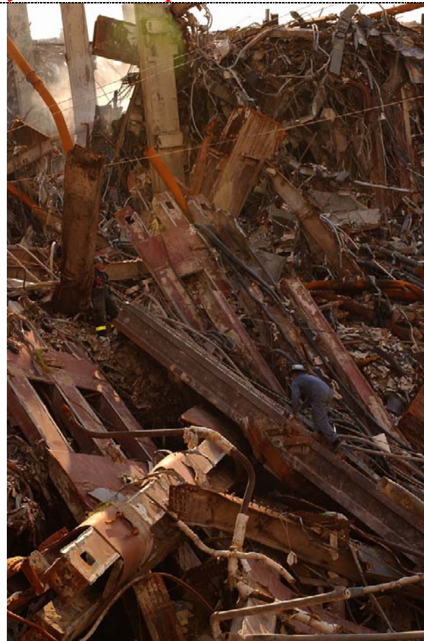
Figure 94. Original photo. It appears that pipes either rusted a lot or not at all.
