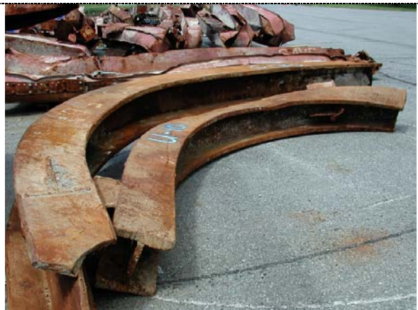
Figure 114. I-beams deformed in the wrong direction. This deformation is inconsistent with overload.
