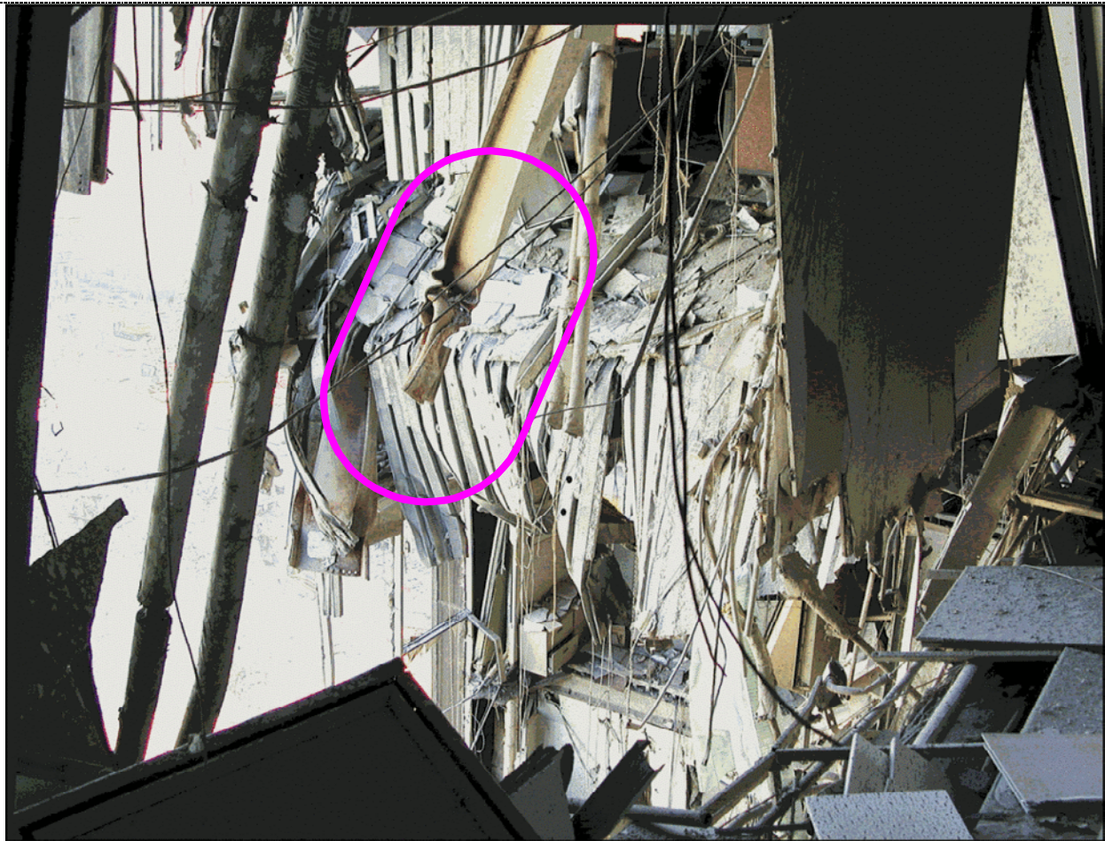
Figure 6-10 Area of collapsed floor slab in bays between C-8, E-8, C-7, and E-7, from the 15th floor.
