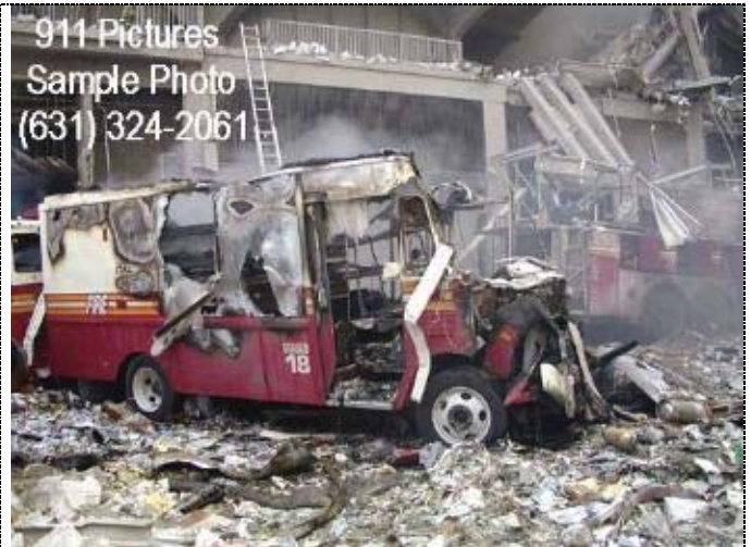
Figure 154. Hazmat vehicle on West Street, in front of WTC6, victimized by DEW on 9/11/01. Note similarities to Figure 153.
