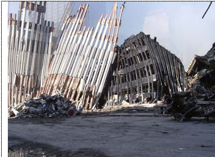
Figure 149. These WTC beams (wheatchex) stabbed into the street without buckling.
