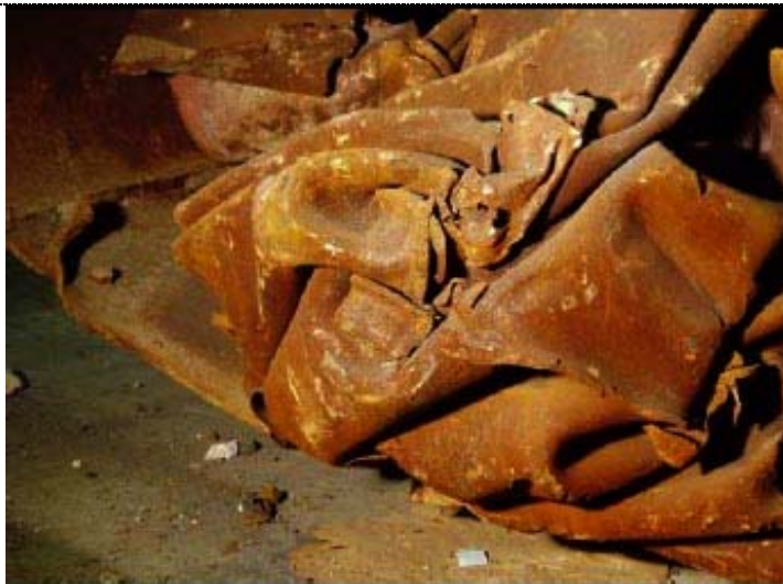
Figure F-A-2c: Collapsed part of Column 210.
